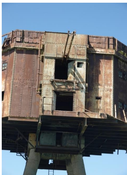
Army Forts Crane Hoist Operative Hatch to right of top doors
