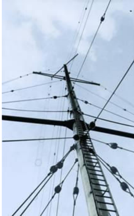
270 mast (collection Peter Messingfeld)
