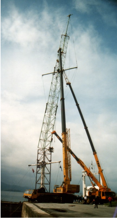
Putting the mast on the MV Nannell (Photo: Archive Hans Knot).
