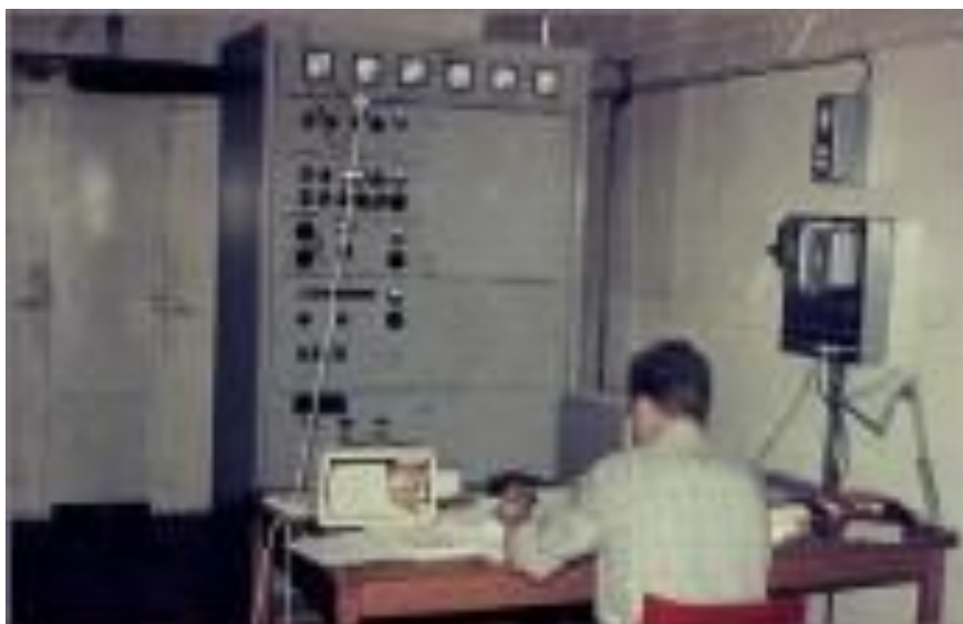
Siemens transmitter on Lucky Star Photo: Soundscapes
