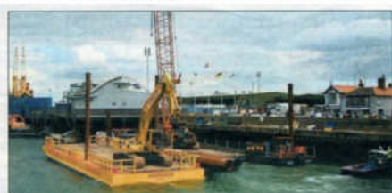
BOOST: Piling work begins for new moorings in Harwich Photo: CONTRIBUTED
