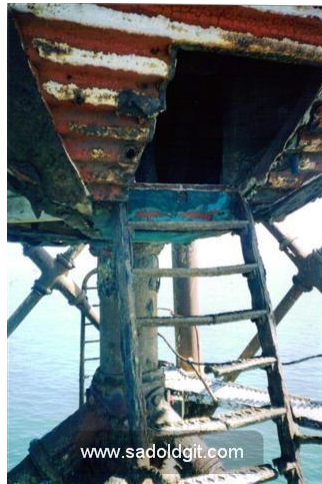
From left to right - more good shots from different view points. The picture below shows the rusty ladder up to the entrance hatch.
